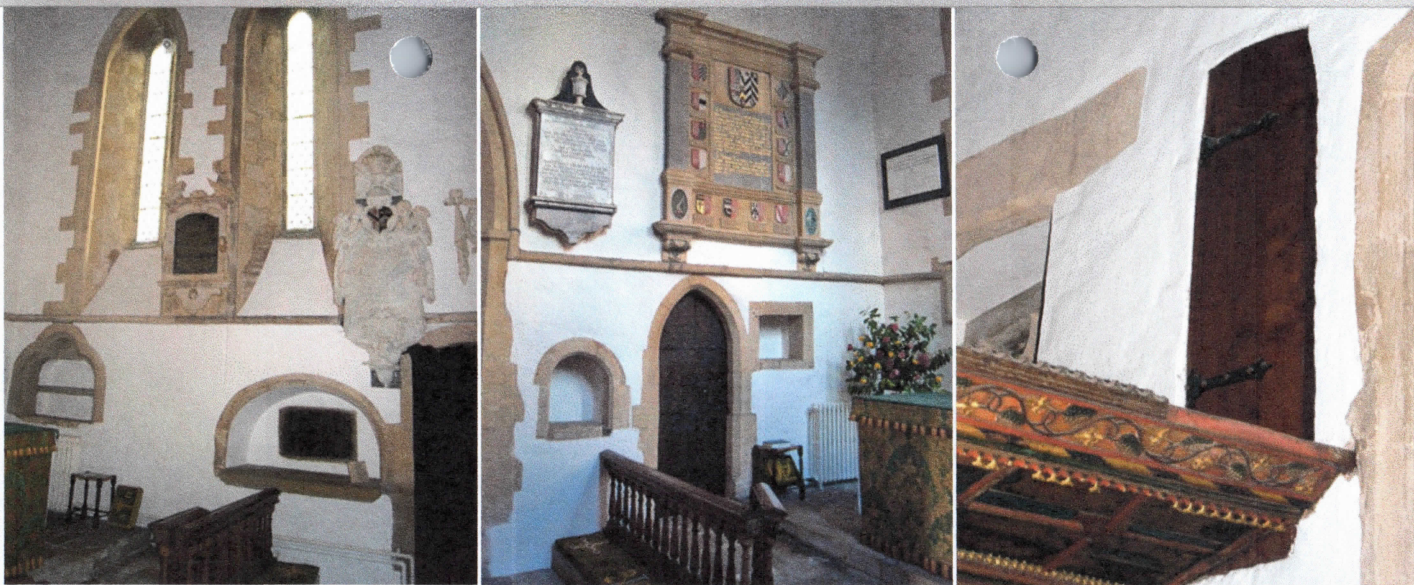
Left: The north wall of the chancel with the lancet windows that so definitively point to early English provenance. Note the brass in the recess to the left of the priest's door. Pevsner suggests this may have been an Easter Sepulchre but they are usually on the north side. Centre: The north wall of the chancel. Is one of these recesses Pevsner's easter Sepulchre? Above the monument you can see the head of a lancet window blocked by the building of a vestry on the other side Right: On the southern side of the south aisle is this comparative rarity: a still functioning rood screen door. How many empty rood stair doors are there in England? Note the fine decoration on the screen itself.
