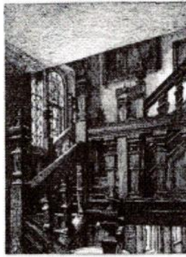
Dinton Hall: The Staircase
